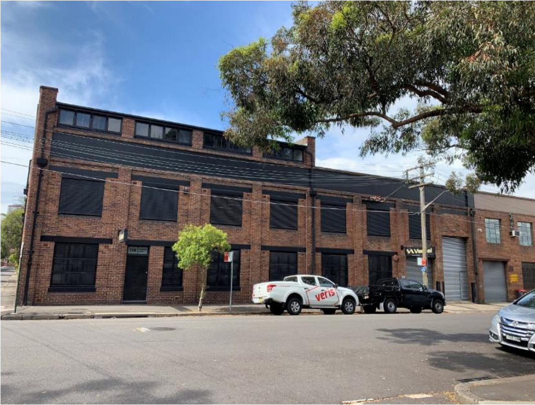
Figure 17 Industrial warehouse building at 116 Wellington Street
