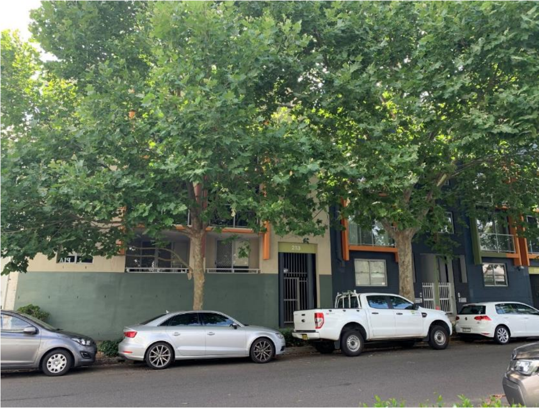
Figure 13 Private strata residential buildings on Cope Street
