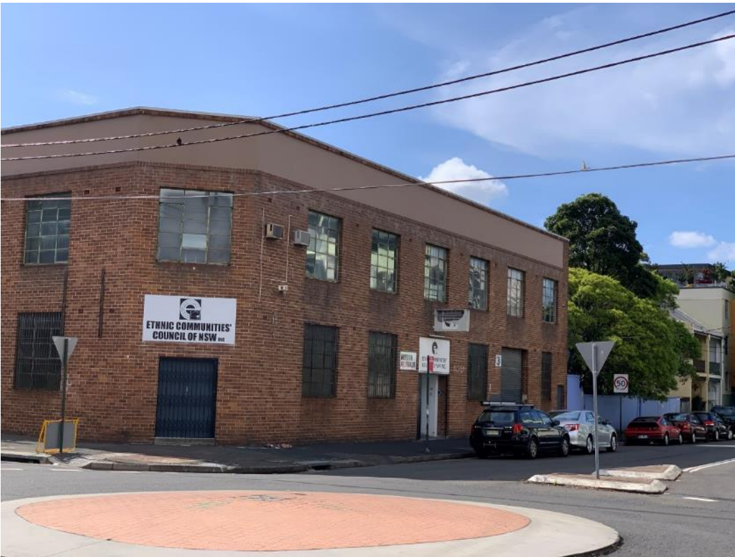
Figure 16 Commercial office building at 221-223 Cope Street
