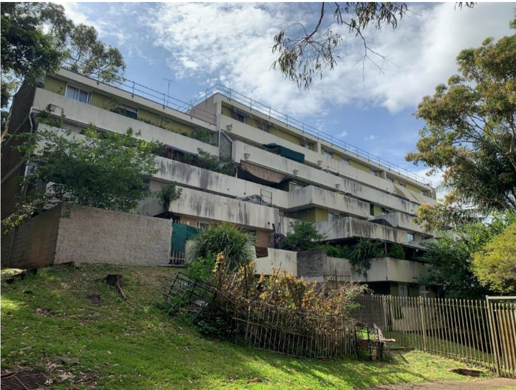
Figure 9 The Dobell building, rear facing John Street
