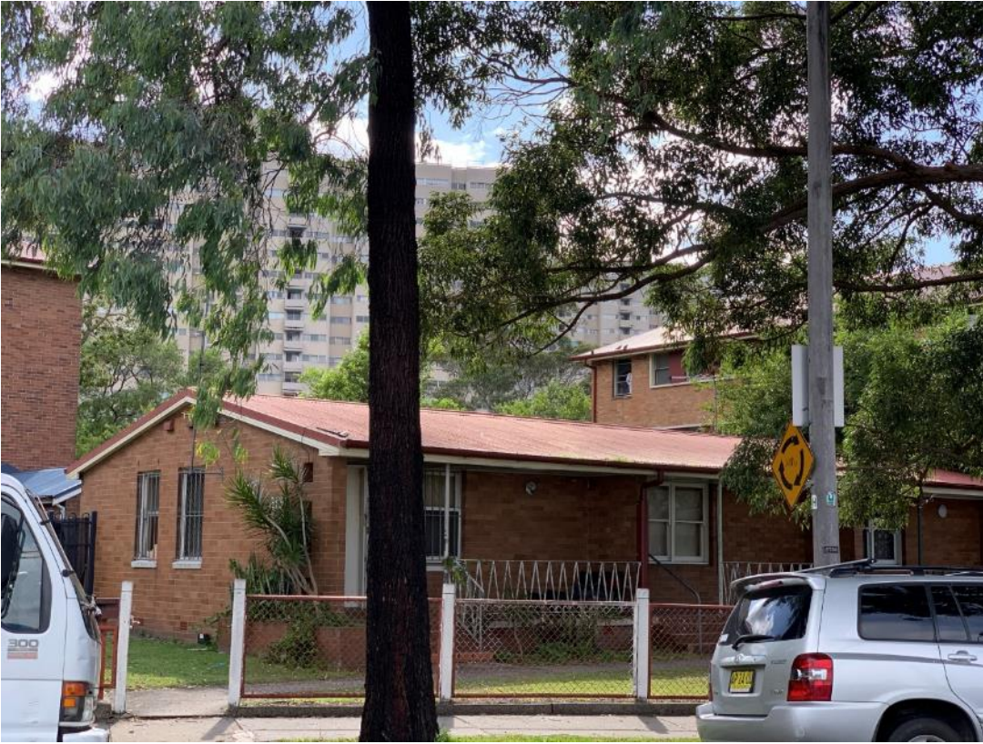
Figure 5 An example of a single storey cottage on the site
