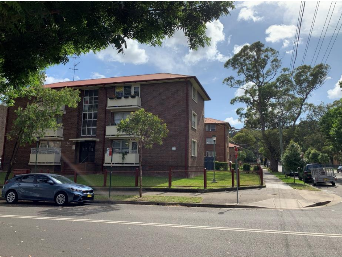
Figure 4 An example of a three-storey walk up apartment building on Cope Street
