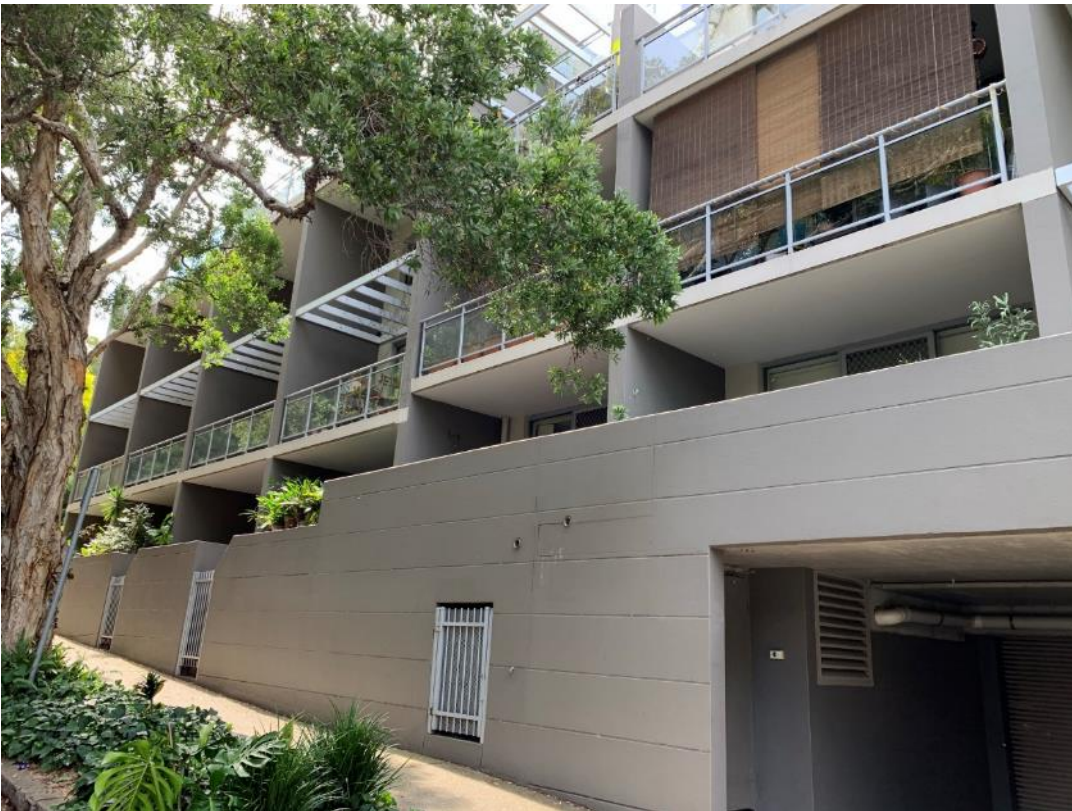
Figure 14 Private strata residential building at 110 Wellington Street
